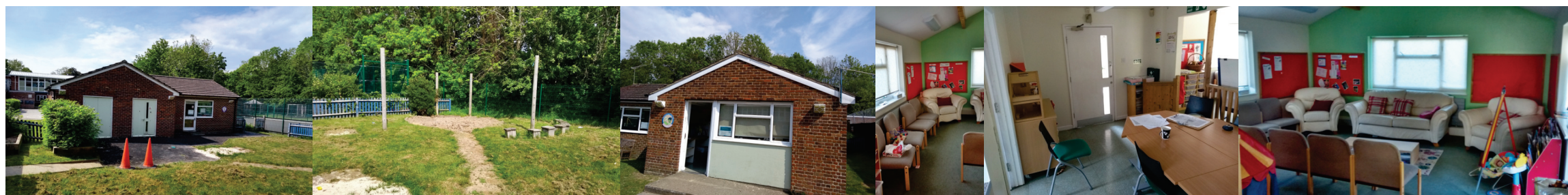
Existing Former Community Building, Woodcot Primary
